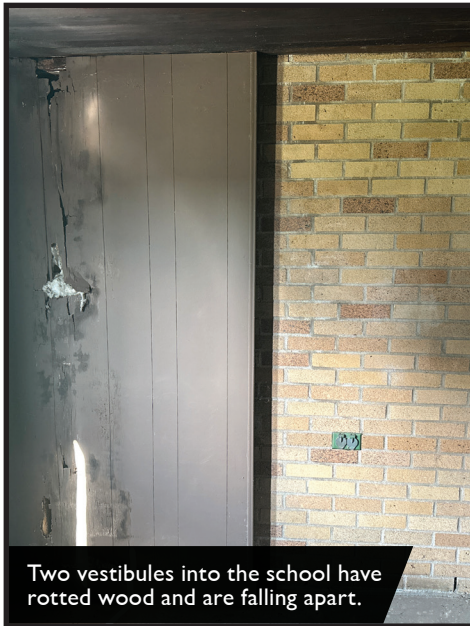
Original doors that were installed in 1957 with wood casework are failing and many do not meet current ADA code requirements.
