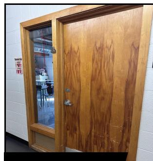
Original doors that were installed in1957 with wood casework are failing and many do not meet ADA code requirements.
